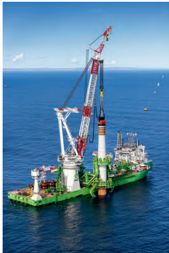
Vibro-pile installation of Moray West foundation
