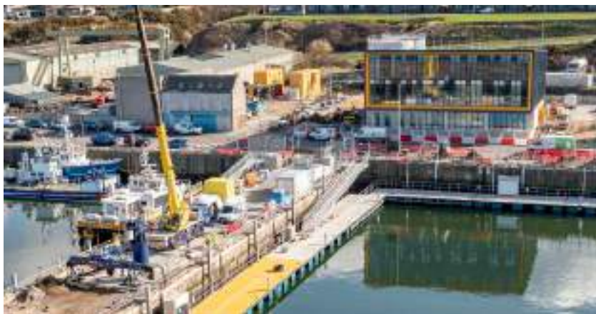
Operations base in Buckie during construction
