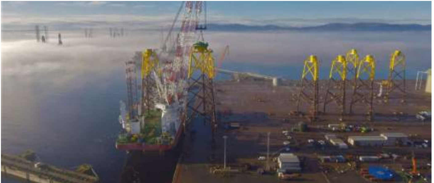
Moray East jackets marshalled at Port of Nigg being loaded onto the installation vessel
