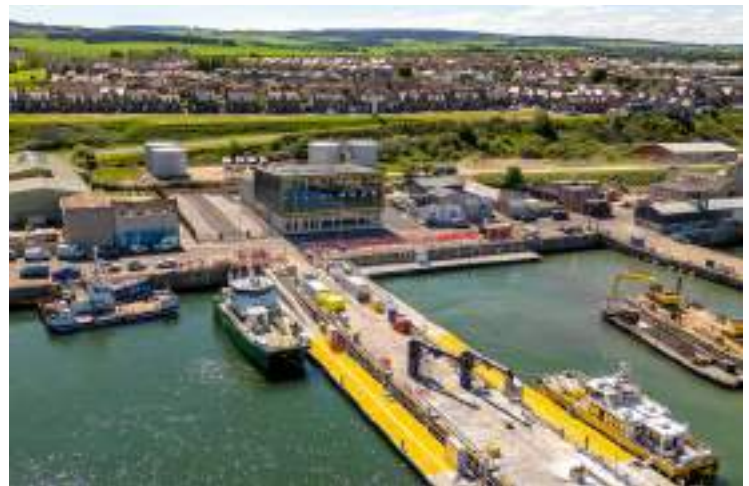
Buckie O&M Base and harbour upgrades, June 2024
